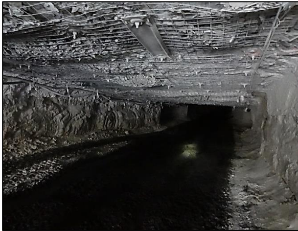
P8 Mine Underground Drive
