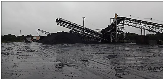
P8 Mine Surface Minesite Infrastructure
